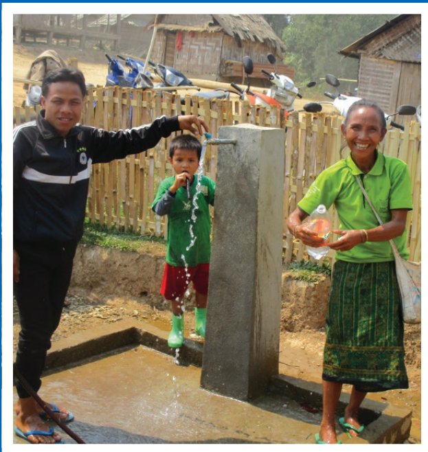
Finally running water in the village.
