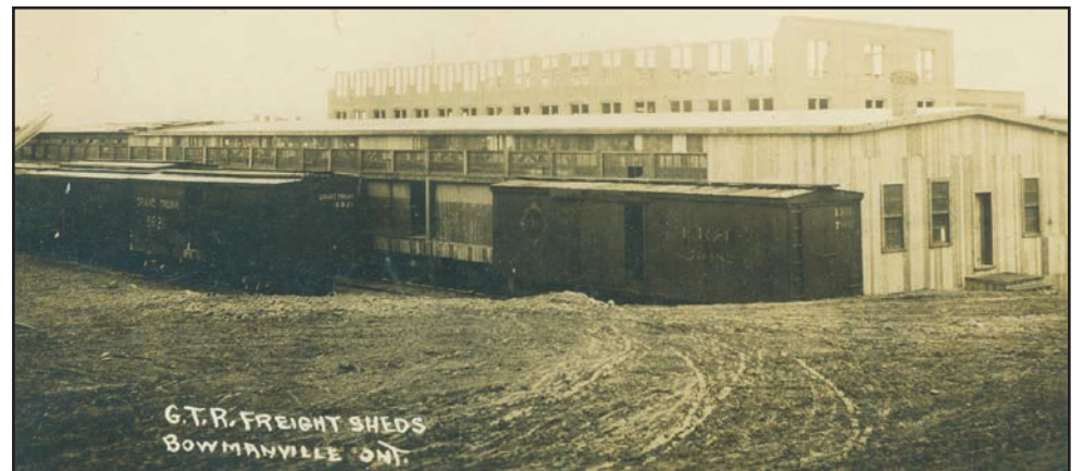
Grand trunk Freight Sheds at the Goodyear Plant. This is where the spur line from the Grand trunk Line (today's Canadian National) ended. It came up from the main line, along the west side of Hunt Street, and into the Goodyear factory complex. The line was taken up a few years ago. A cement whistle post (a sign to tell the engineer to blow his whistle before crossing the Baseline) was relocated to the backyard of the Bowmanville Museum. In this c. 1910 photo part of the Goodyear Factory is still under construction.
