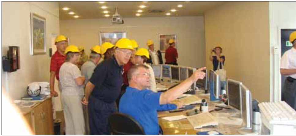
Councillors and Members of Staff from Clarington and Durham Region inspect the control room of an Energy-from-Waste facility during the July 2007 European Tour. Computer Control Room Manager explains to Councillor Nester Pidwerbecki how the stack emissions are controlled, monitored and recorded on a 24/7 basis to ensure the facility operates within the European Union Guidelines (above). Control Room Flow Chart explaining to visitors the various stages required to remove energy from garbage (below).
