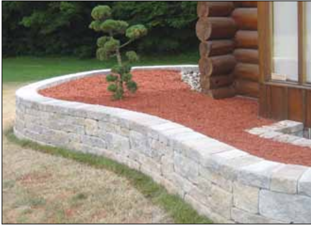
Beautiful retaining walls add curb appeal as well as function when properly constructed. Be sure to follow basic guidelines to create a lasting project.
