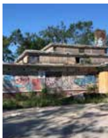
1 of 6 historically designated buildings (photo taken August 14, 2019)
