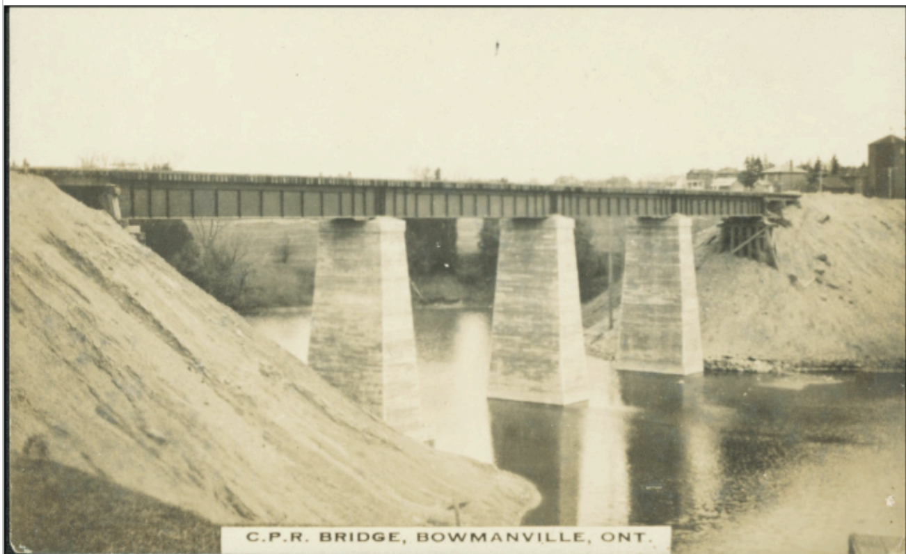
The Canadian Pacific Railway Trestle over Vanstone's Pond was considered quite an engineering feat in its day. This photo shows it just after completion around 1912. To the extreme right a water tower, used to provide water for the steam locomotives, can be glimpsed.
