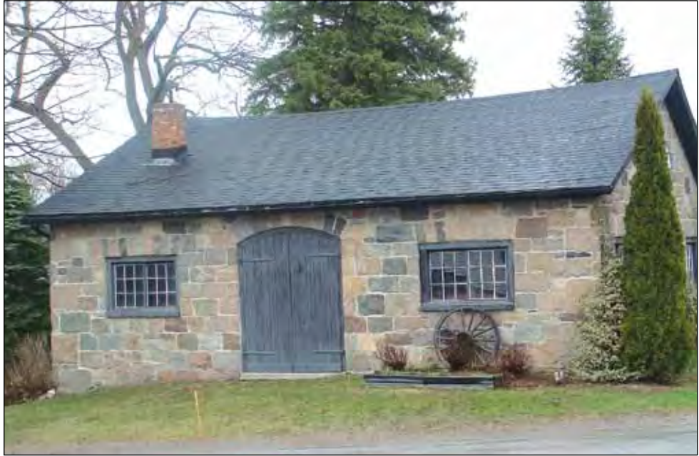
Tyrone Blacksmith Shop - This unique structure is one of the architectural gems of Clarington. Built in 1860 for blacksmith George Emmerson, it is best remembered for his apprentice, Robert McCullough, who ran the shop from 1895 to 1950.
